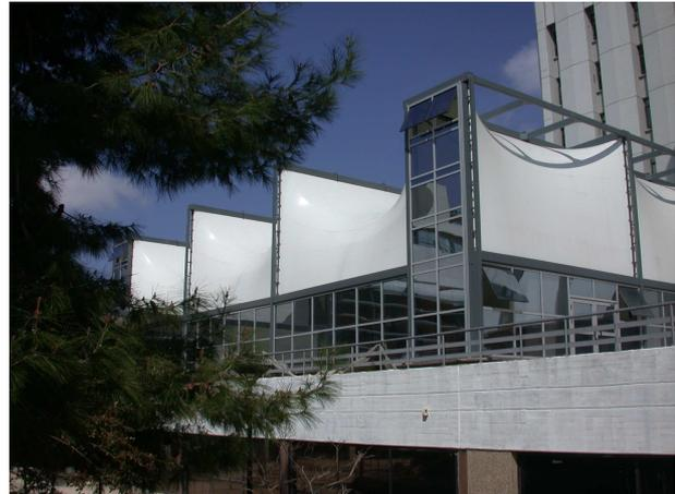
*Fig. 4 – The Amado membrane roof structure – the overall orthogonal assembly composition of rigid-edge membrane units.*
