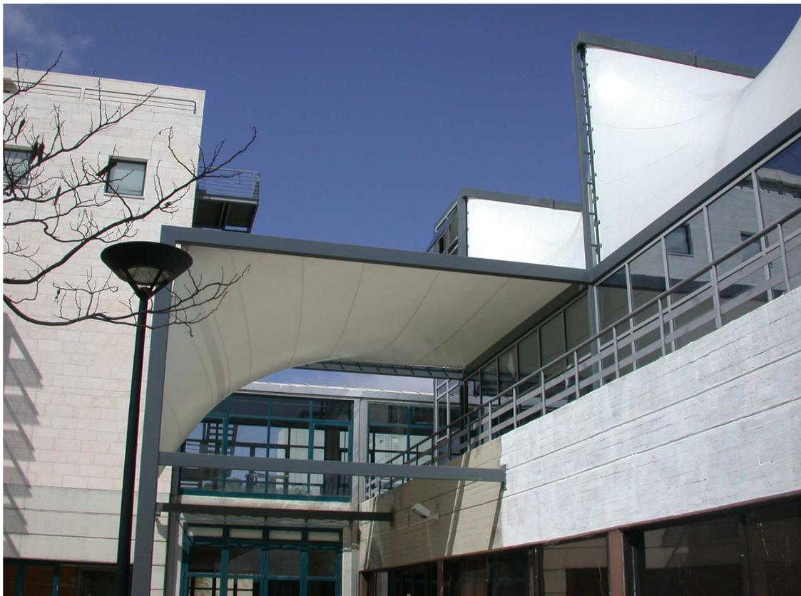
*Fig. 12 – Amado Roof; Exterior view of the rigid-edge orthogonal composition of membrane units and glazed facades.*
